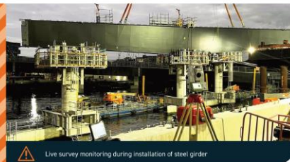
Live survey monitoring during installation of steel girder
